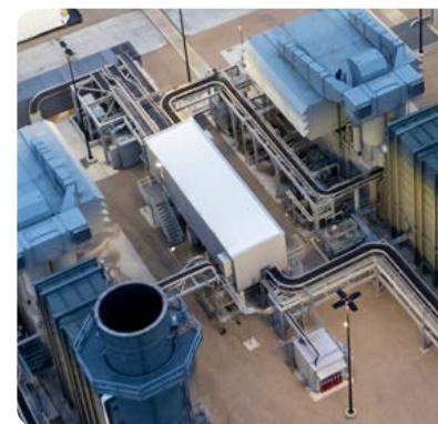
**PDC** enables operating two generating units and includes a custom-built enclosure, control panels, electrical equipment, and cabinets.
