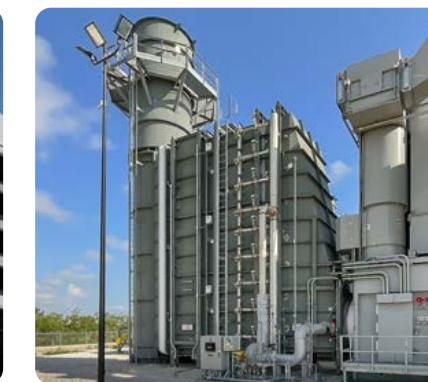
**Emissions control system**, with exhaust stack, ammonia system, and selective catalytic reduction / carbon monoxide reduction (SCR/COR), reduces greenhouse gas by 90 percent or more.
